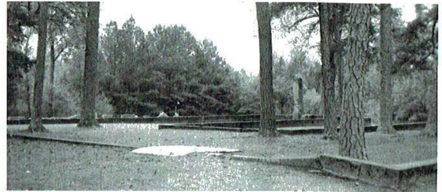
The foundation of the girls' dormitory.
