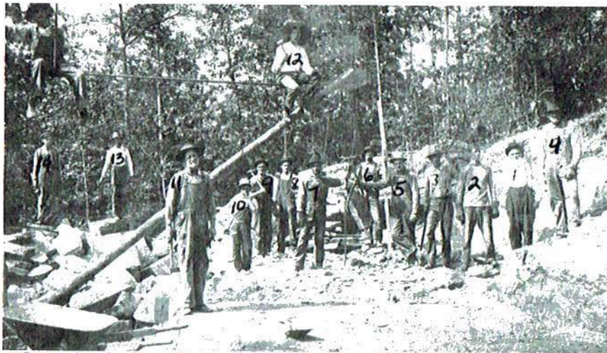
Quarrying the donated stone from the property of A.J. Hogue, to be used in the construction of Flat Rock High School's Administration Building are:
